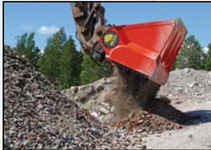
Crushing bricks / black top asphalt
