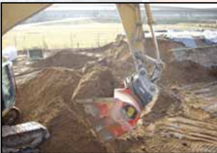
Stabilising foundation layers
